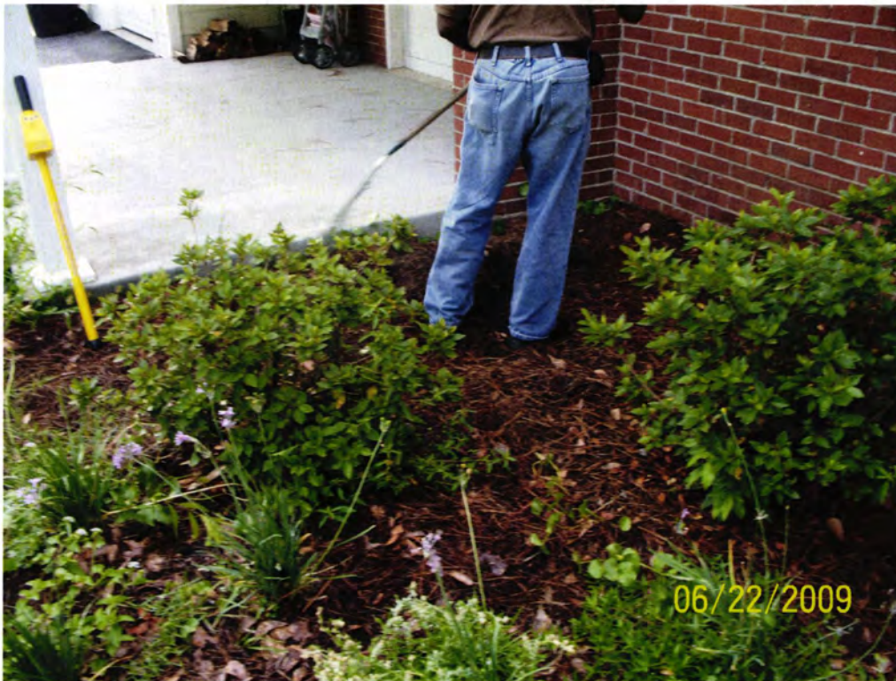
Picture 1: Location of UST 1129Iris prior to excavation.
