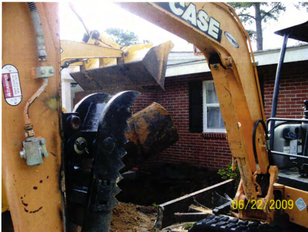
Picture 2: UST 1129Iris during removal.
